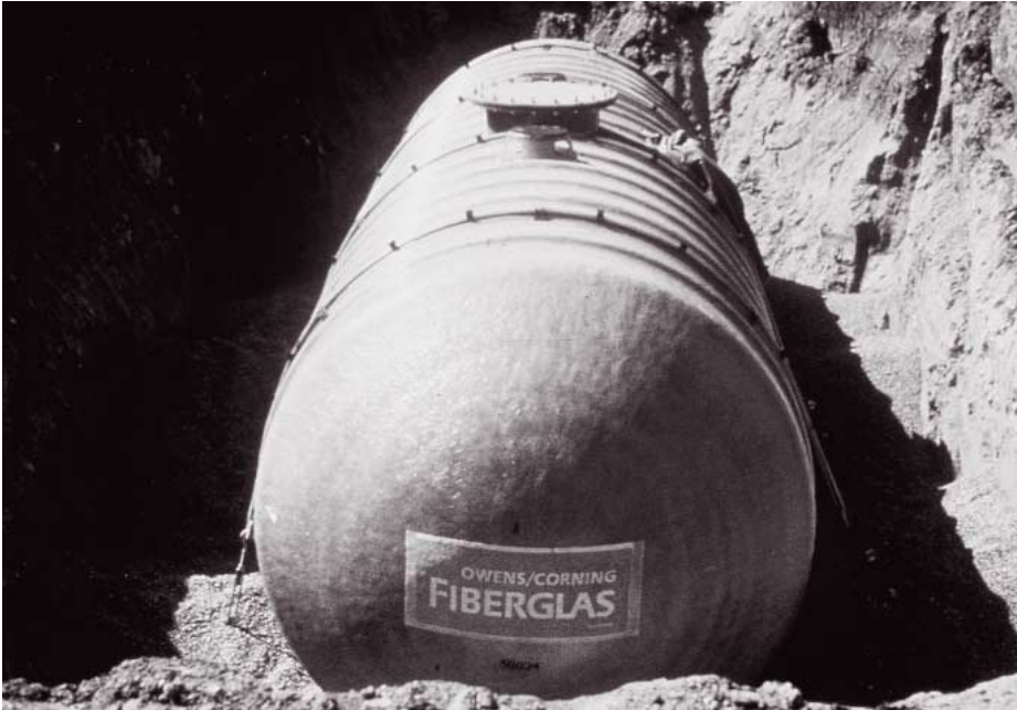
New installation of a fiberglass underground tank.
