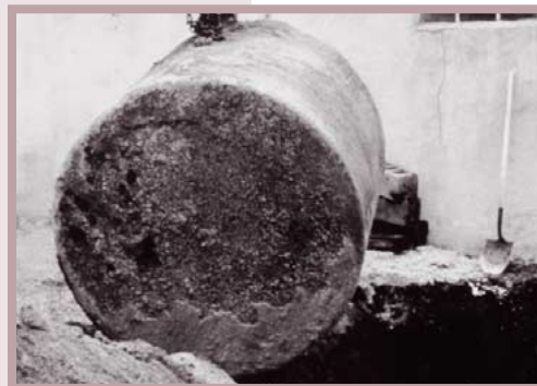
Removing a corroded tank
